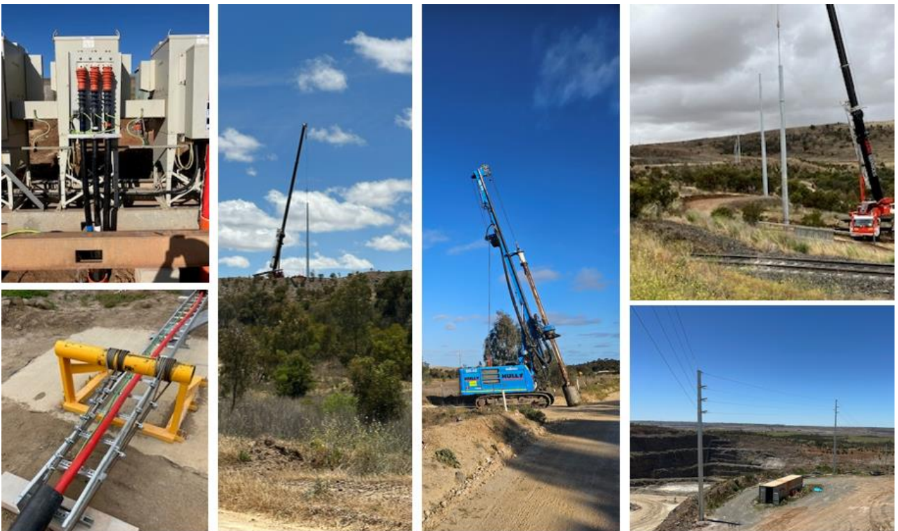
Figure 6 Installing the overhead powerlines from the main switchyard to the underground operation
